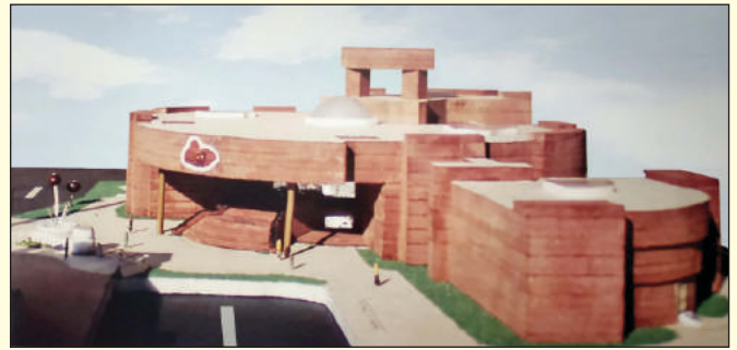
Fig. 16 : Front view of the building
