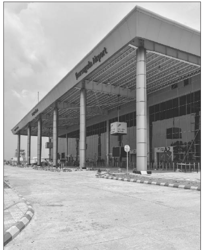
Extended Canopy Around The Terminal
