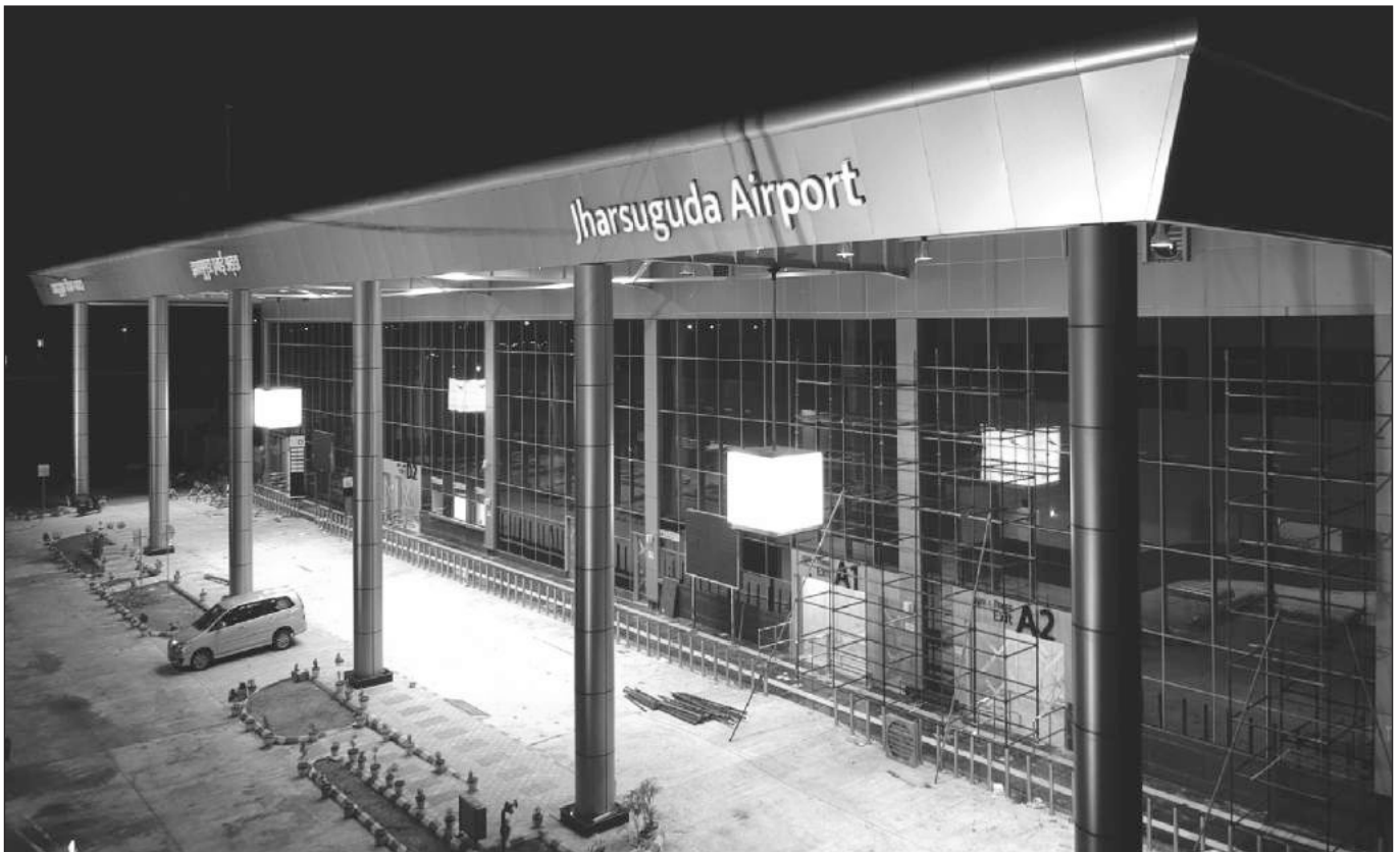
Reflective Façade With Highlighted Entrance
