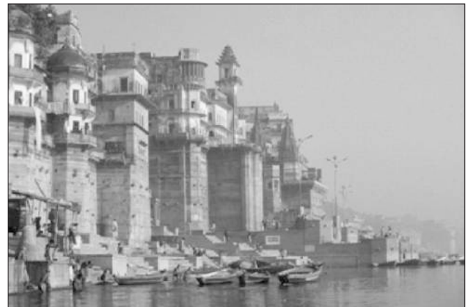
Fig. 1 - The design language with the lower floors solid and upper floors porous to resist the thrust of the river when it floods.
